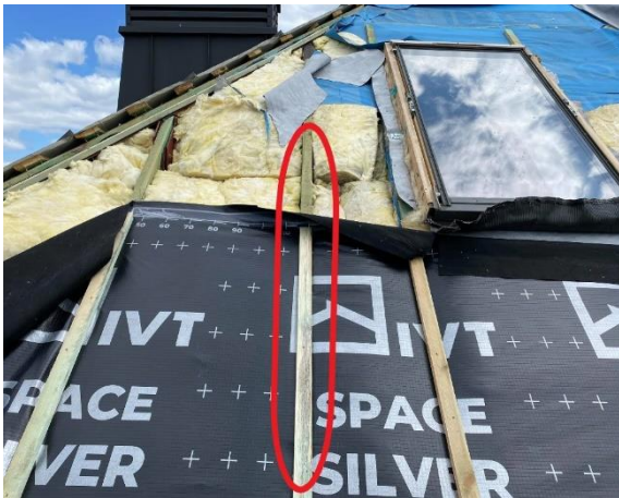
Fig. 3c. Counter battens (counter batten marked in red) and black wind resistant membrane under counter battens [7].
