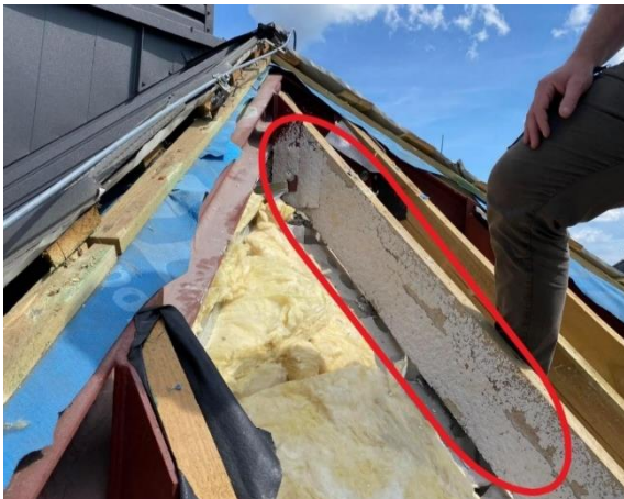
Fig. 3e. Timber roof rafter (marked in red) [7].
