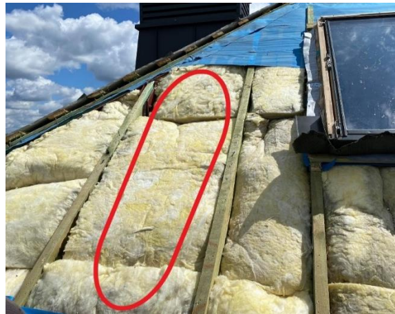
Fig. 3d. Mineral wool (marked in red) [7].
