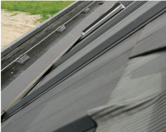
Fig. 3a. Roof covering – standing seam coated steel roof panel [7].
