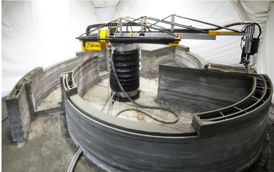
Fig. 1. Apis Cor 3D printer (8.5 m x 1.6 m x 1.5 m) [Walasek M., 3d.edu.pl, 2021].
