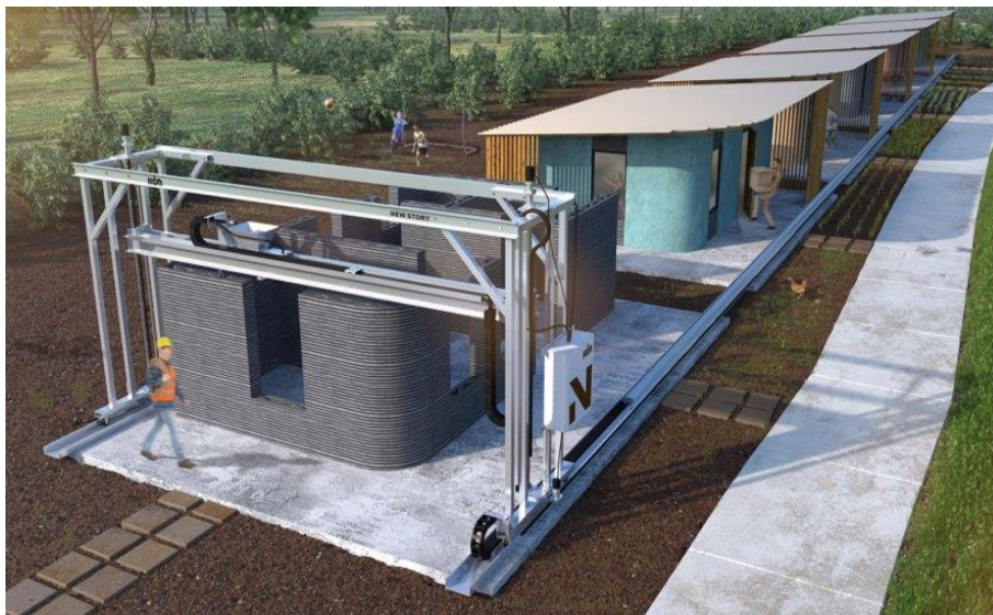
Fig. 2. Vulcan 3D printer (11.5 feet high, 33 feet wide) [Walasek M., 3d.edu.co.uk, 2021].
