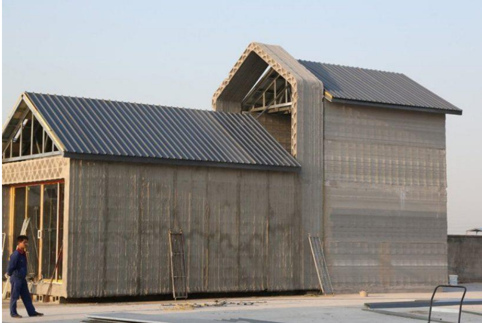
Fig. 9. 3D printed houses by WinSun in China [PlanRadar, 2022].
