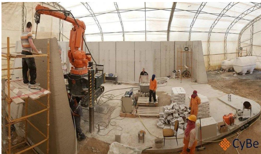
Rys. 4. Drukarka CyBe Construction CyBe RC 3Dp, CyBe R 3Dp [Walasek M., 3d.edu.pl, 2021].
