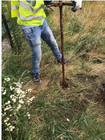
Fig. 5. Overall view of the soil borehole made using a hand auger.
