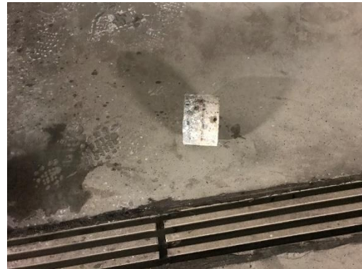
Fig. 2.2. Overall view of the borehole in the underground garage floor.
