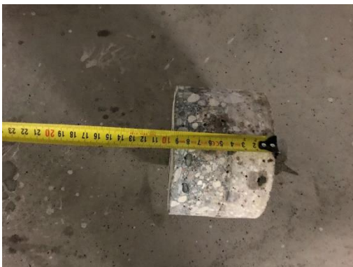
Fig. 2.3. Measuring the thickness of the borehole in the underground garage floor: 9.5 cm.
