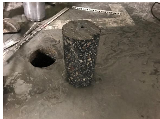
Fig. 2.4. Overall view of the borehole in the underground garage foundation slab.
