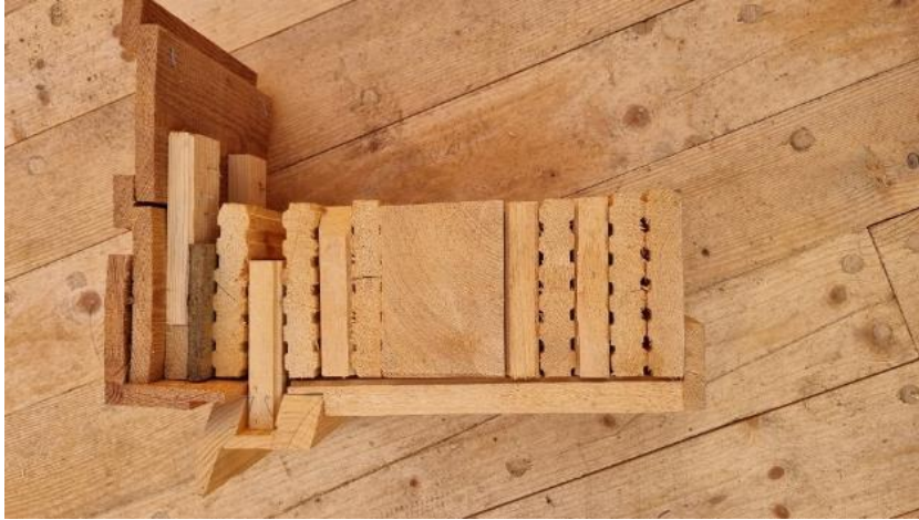
Fig. 21. Cross-section of the external wall (own photos).
