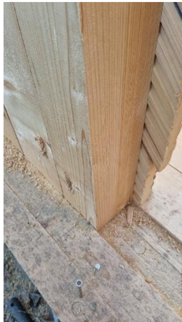
Fig. 20. Supporting the outer wall on the load-bearing board (own photos).
