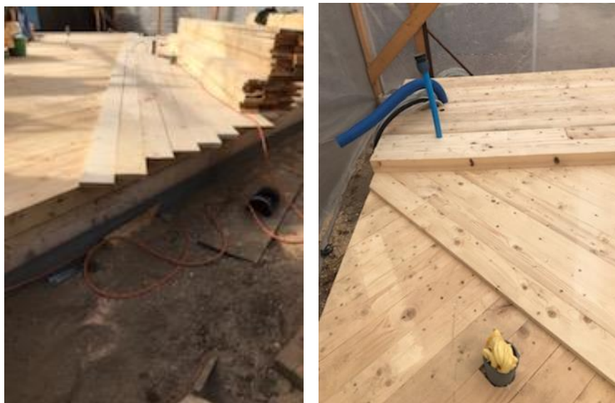
Fig. 16, 17. Laying layers of wooden board (own photos).
