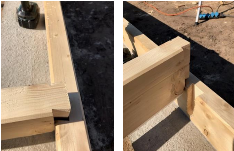
Fig. 10, 11. Dovetail connection in the plate (own photos).
