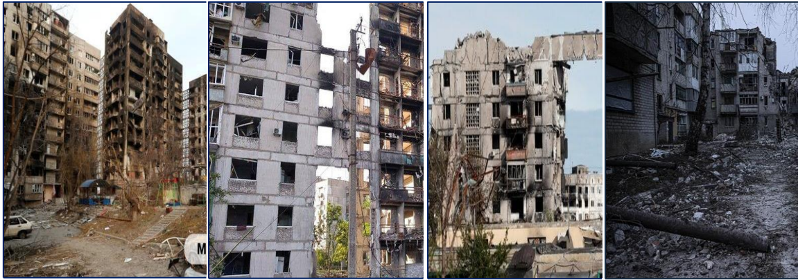
Fig. 11. Large-scale destruction of buildings in Ukrainian cities as a result of Russian shelling and bombing
