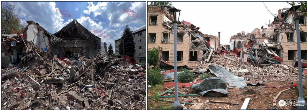
Fig. 10. Construction debris that requires recycling for secondary use
