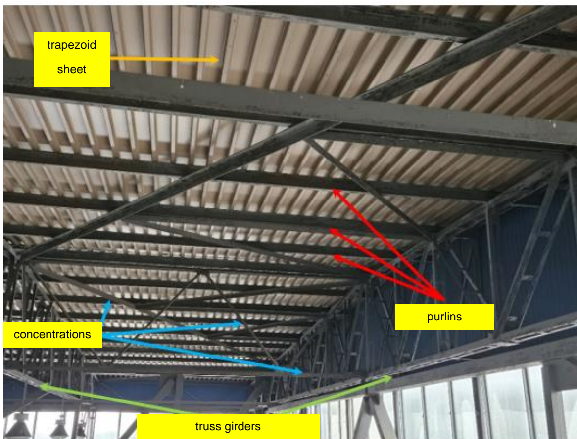
Fig. 1. The hangar roof structure.
